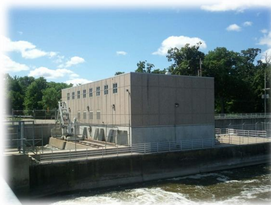
2 Megawatt Hydro Facility
